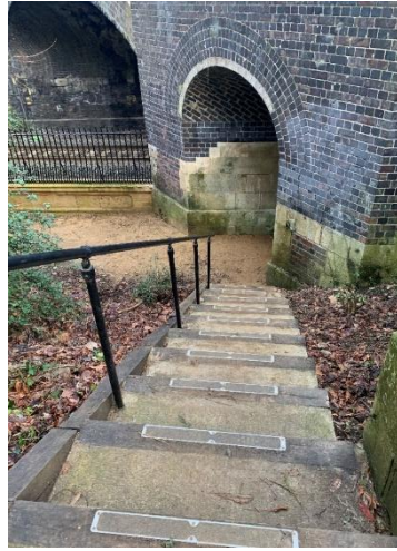
Step access to the railway line
